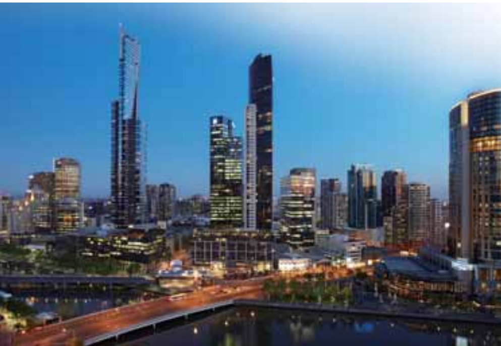
▶ CitiPower supplies electricity in Melbourne's CBD and inner suburbs.
