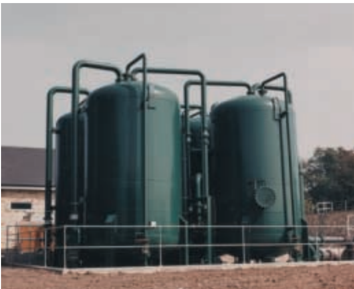
Cambridge Water scores top rank from Office of Water Services for operating efficiency.
