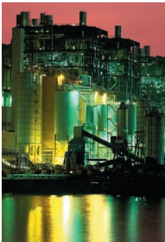
Lamma Power Station at night showing important environmental protection facilities: ash silos (foreground) and boilers fitted with low NOx burners (background).
