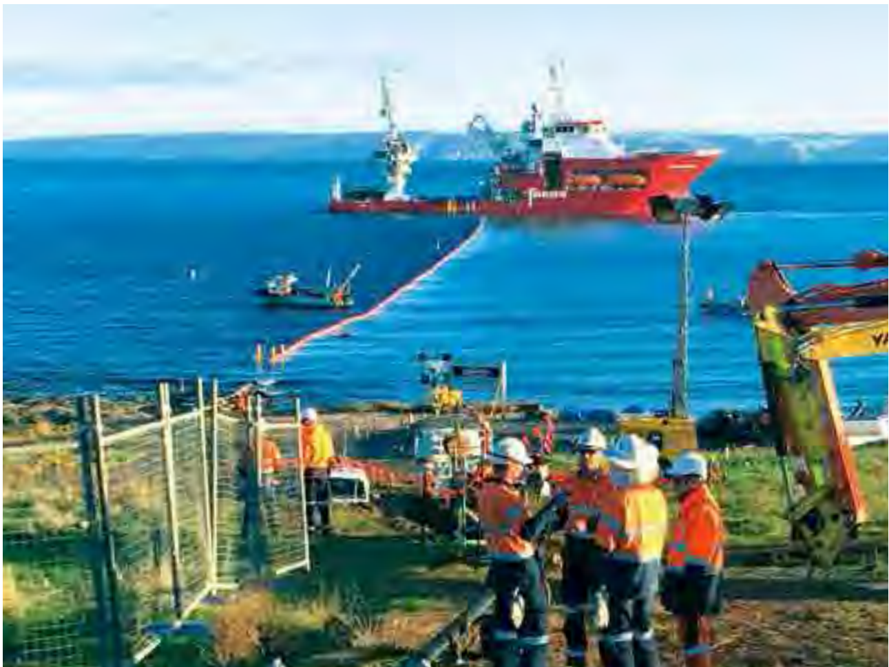
The replacement of the undersea cable connecting Kangaroo Island to the South Australia electricity distribution network was successfully installed.
