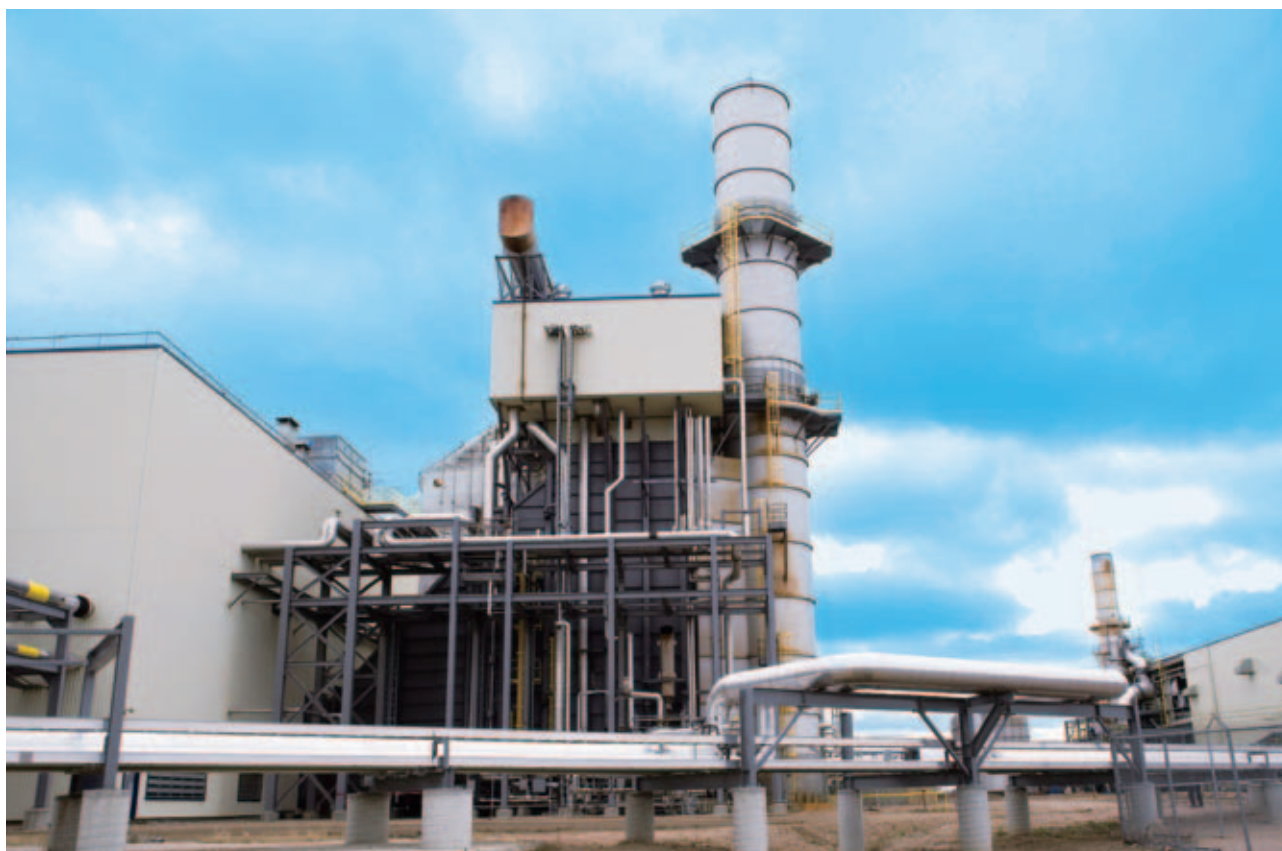
Canadian Power has a total generating capacity of 1,368 MW that can supply over 500,000 homes.
