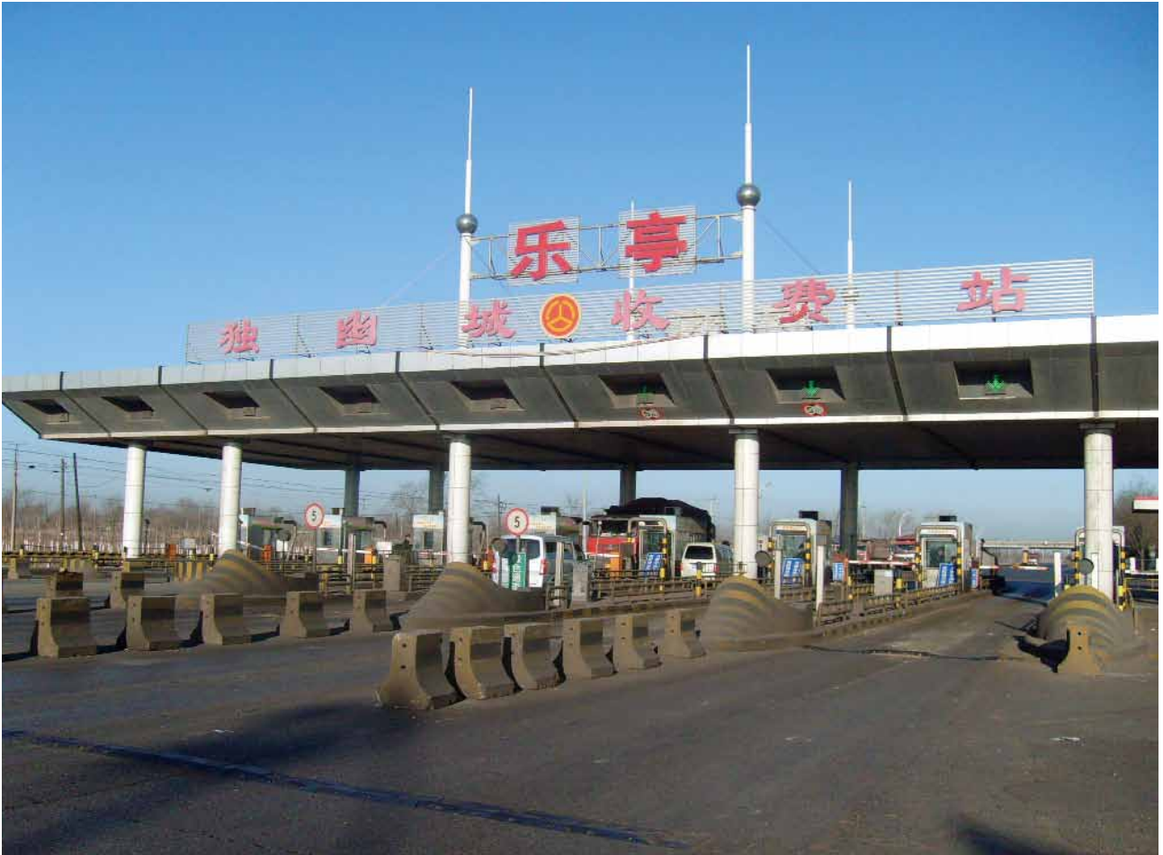
■ CKI has a shareholding in six toll roads and bridges across Mainland China.
