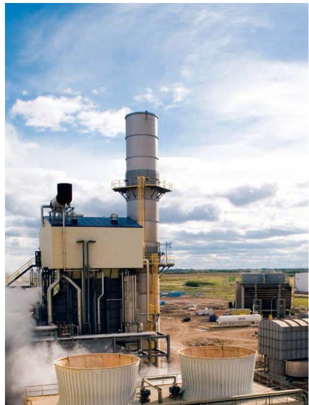
The acquisition of the Meridian Cogeneration Plant has enhanced the Group's portfolio and revenue stream in Canada.
