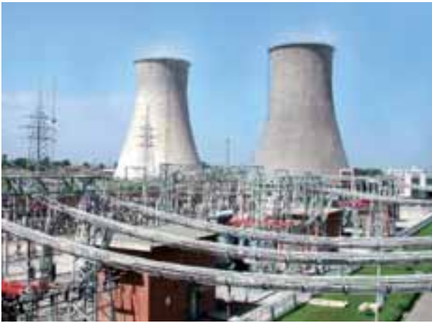
An all-round satisfactory performance was achieved by the Siping Cogen Power Plants in Jilin.
