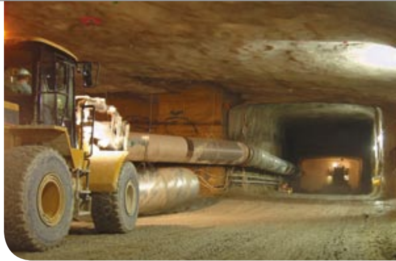
Steady progress is being made on the construction work for the Lane Cove Tunnel in Sydney, Australia.
