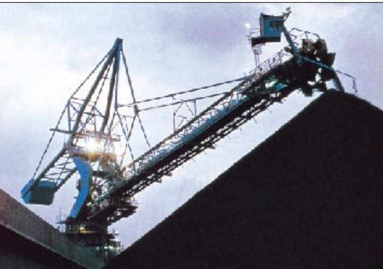
The Lamma Power Station, the only power station operated by Hongkong Electric, has an installed capacity of 3,305 MW.
