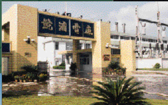
Shantou Tuopu Power Plant
