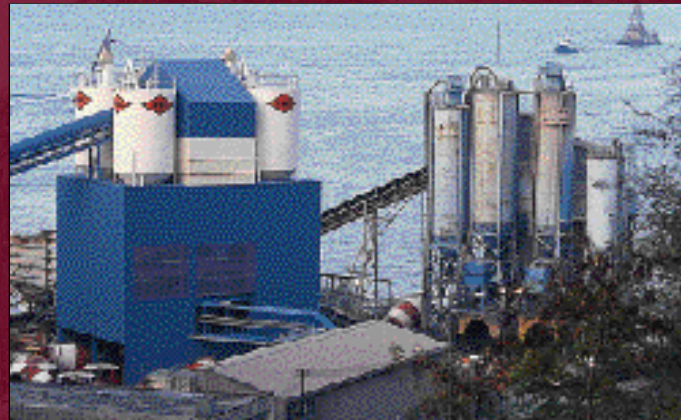
Ready Mixed Concrete, Anderson Asia (below and right)
