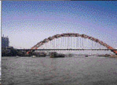
Sanshan West Bridge of the Nanhai Road Network
