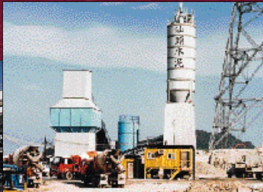
Shantou Cement Plant - under construction
