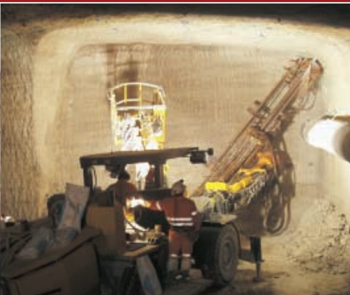
LANE COVE TUNNEL
